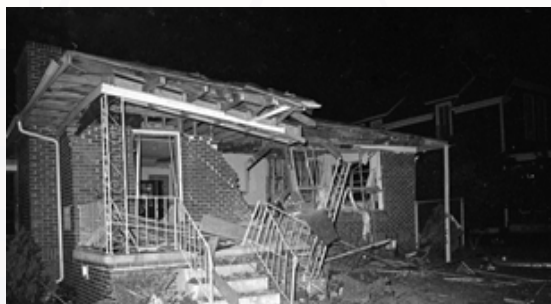
Significant damage to MLK's home
